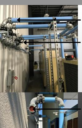
ACF Pipes all compressor discharges up and then down into the system header. This assures liquid water will not get blown downstream and is drained out through drain ports at the lowest point in the system.
